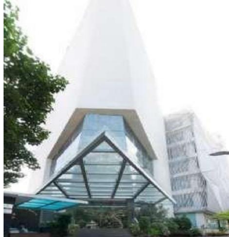
CCIL Bhavan Phase I Upto 6 th floor
