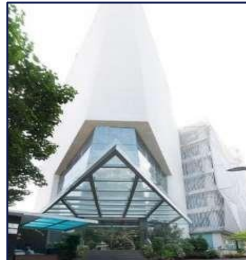
CCIL Bhavan Phase I : Upto 6 th floor
